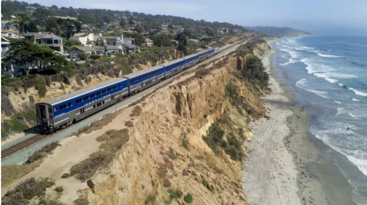
San Diego "Coaster" passes 20 feet from eroding 100' cliff in Del Mar , 2019. Since that time, the cliff has collapsed, shutting down rail service.
